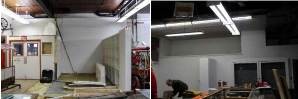
After demolition and re-painting January 2018.
